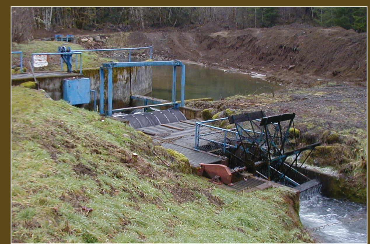
Settling pond and old screen
